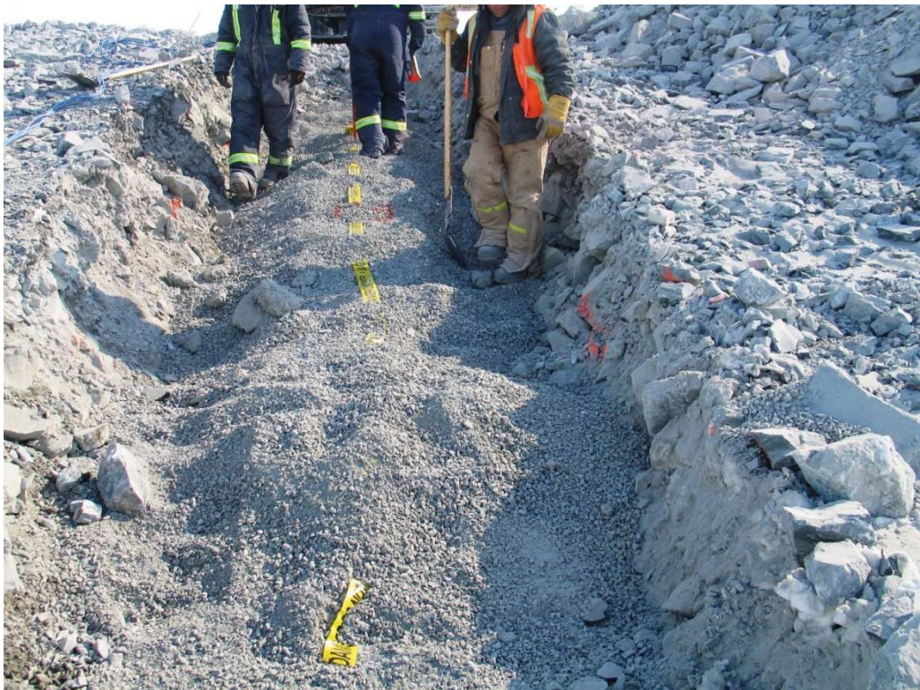
Photo 4: Warning tape placed over final lift crush
