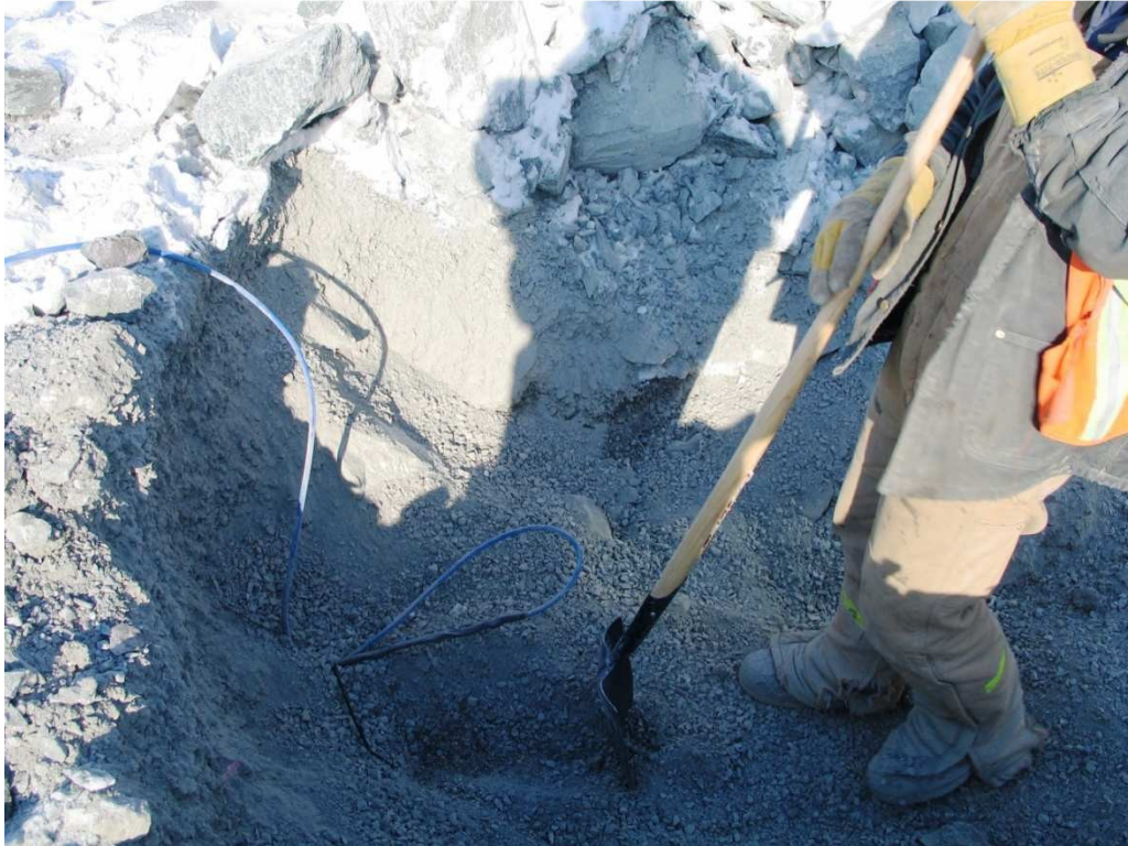
Photo 7: Sta 0+60 Coil in cable ~ 2 feet down.
