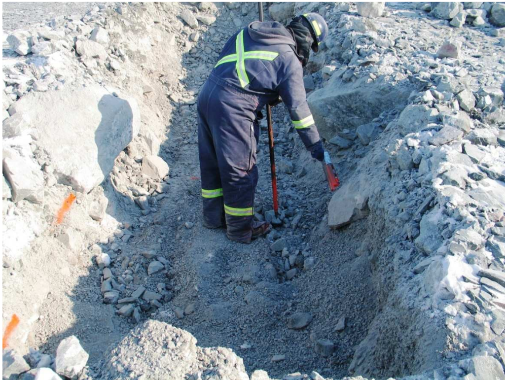
Photo 8: Surveyor marking crush fill levels.
