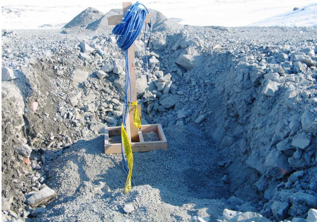
Photo 5: Termination of cables at Sta 0+40
