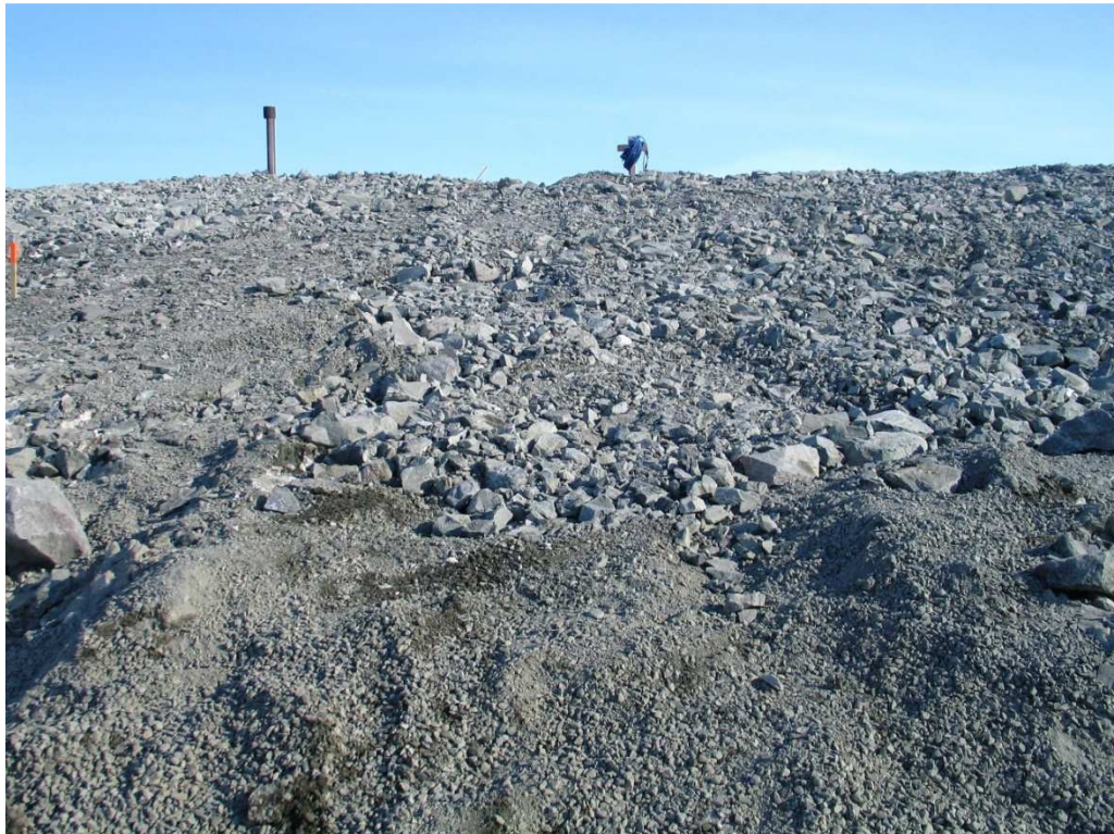
Photo 6: Finished product Sta 0+40. Still to be compacted with 10 ton packer
